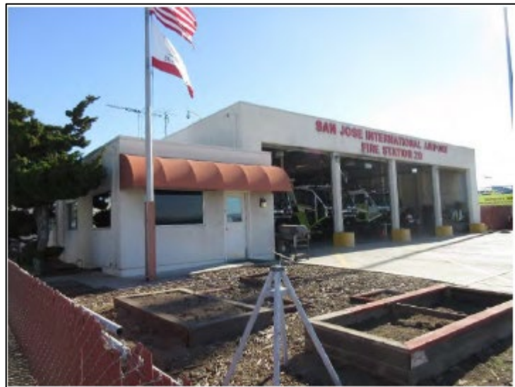
Photo 9. Aircraft Rescue and Firefighting Building southwest elevation, view to the northeast (Photo courtesy of the Evaluation of San Jose International Airport Aircraft Rescue and Firefighting Building Memorandum, 2018)
