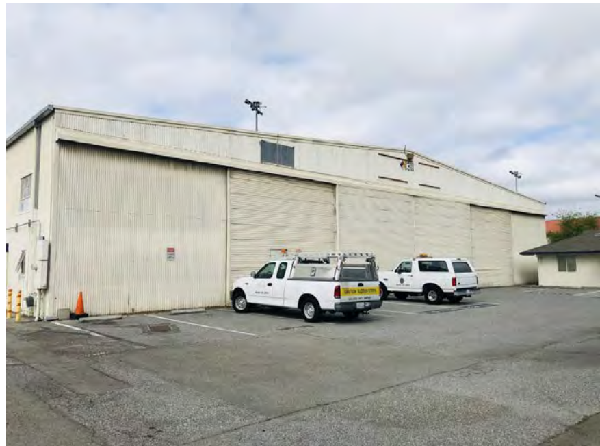
Image 26: Hangar 1311 northeast elevation, view to the west
