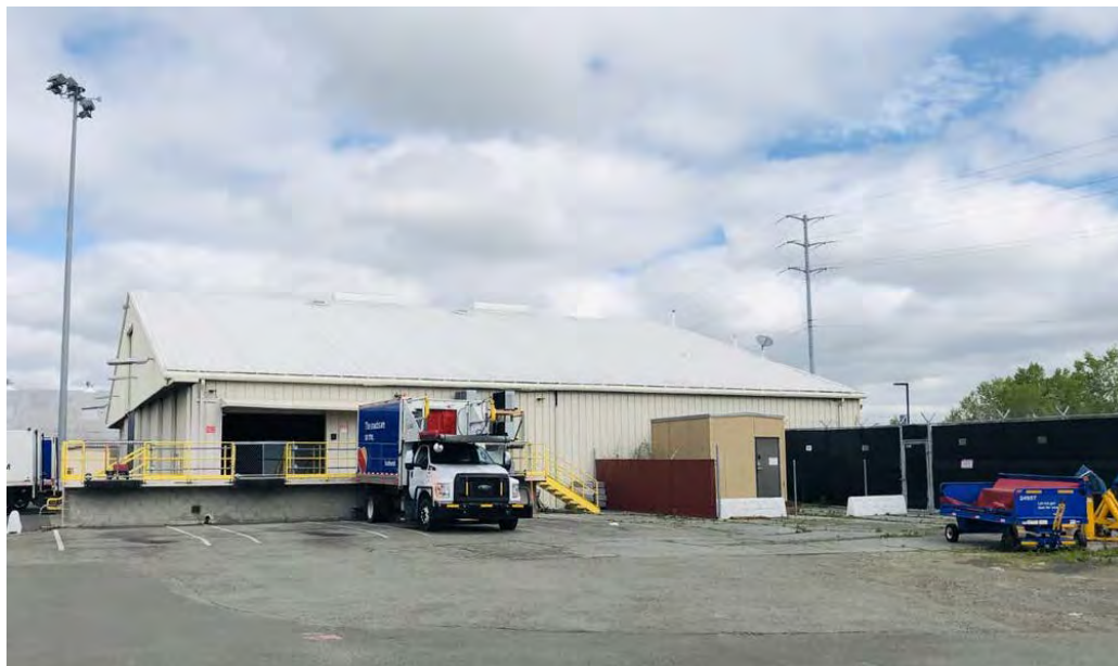
Image 33: Hangar 1239 southeast elevation, view to the northwest
