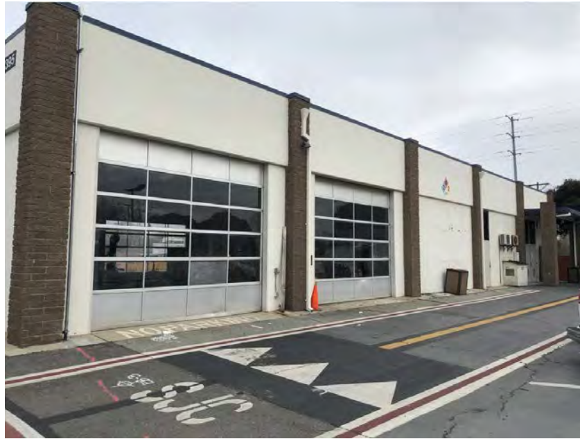
Image 19: Facilities Building (1395A) east elevation, view to the northwest
