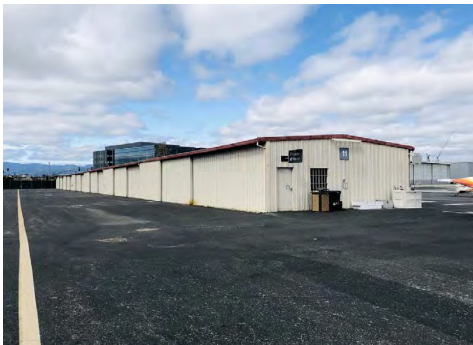
Image 40: Hangar 11 northeast oblique, view to the southwest
