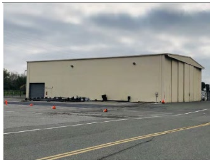
Photo 4. Support Hangar (ACM/Pestana Support Hangar) northwest elevation, view to the east
