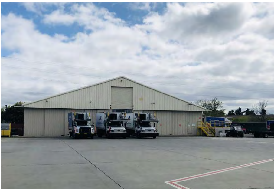
Image 32: Hangar 1239 southwest elevation, view to the northeast
