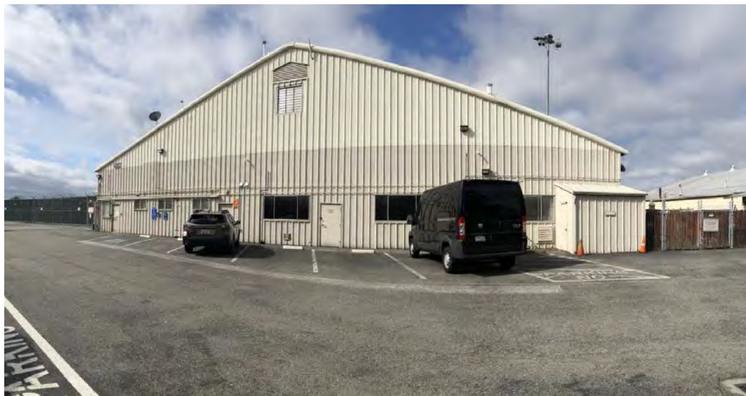
Image 34: Hangar 1239 northeast elevation, view to the southwest
