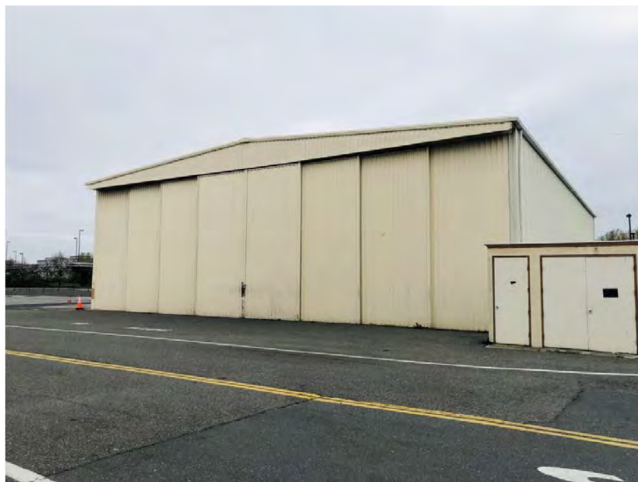
Image 14: ACM/Pestana Support Hangar southwest elevation, view to the north
