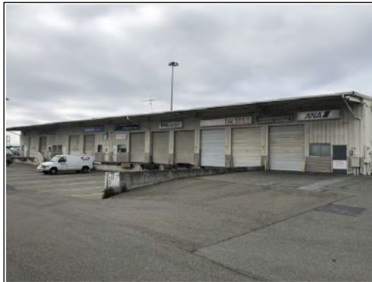
Photo 6. Air Freight Hangar – Belly Freight northeast elevation, view to the south
