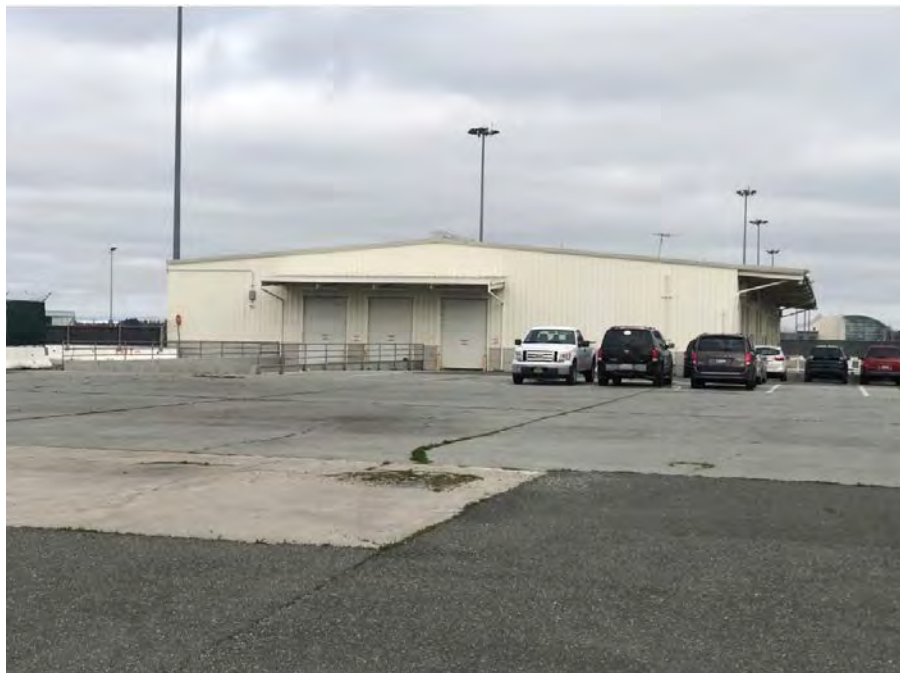
Image 9: Air Freight Building southeast elevation, view to the west
