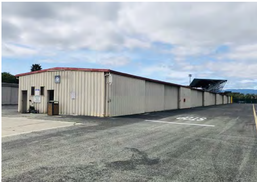
Image 38: Hangar No. 9 northeast elevation oblique, view to the southwest
