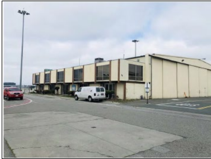
Photo 1. SJPD Hangar (ACM/Pestana) southeast elevation, view to the northwest
