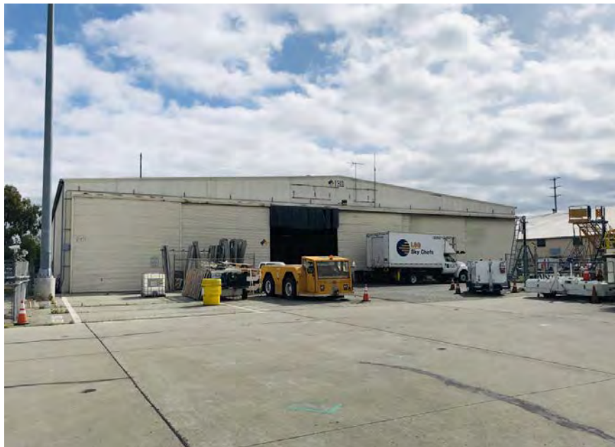
Image 24: Hangar 1311 southwest elevation, view to the northeast
