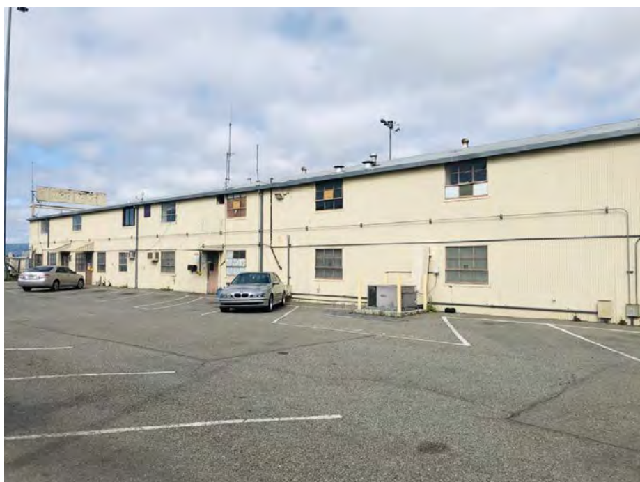
Image 28: Hangar 1277 southeast elevation, view to the west
