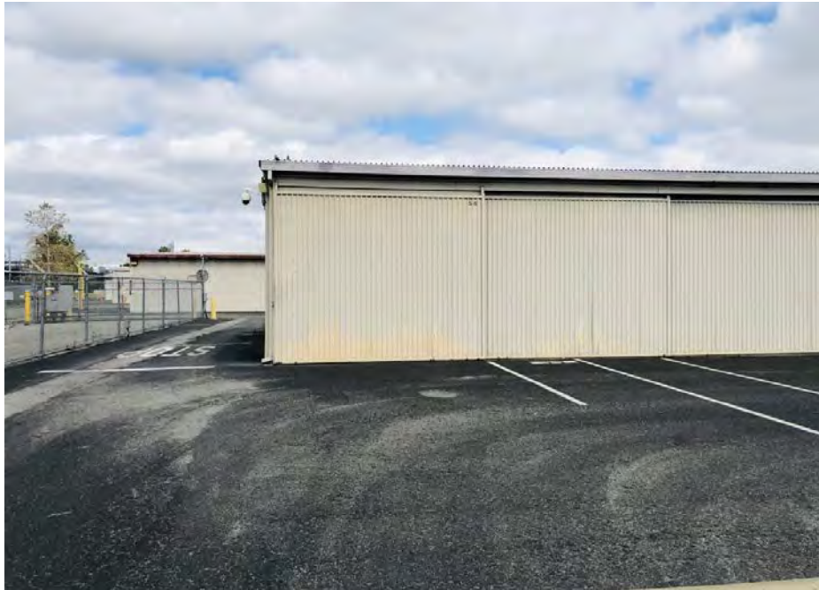
Image 37: Hangar Nos. 8-11 southeast elevations, view to the northwest
