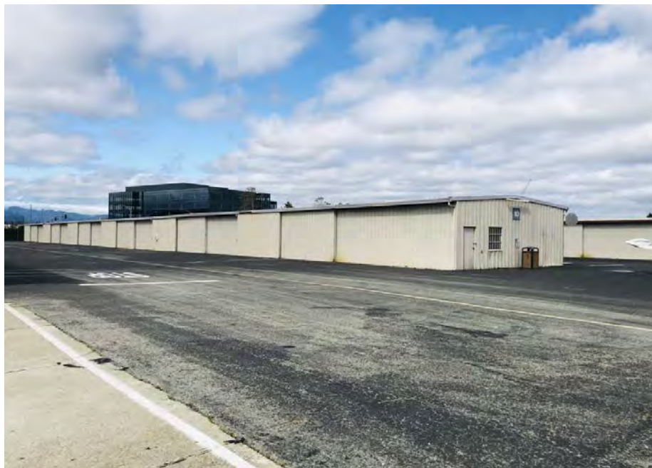
Image 39: Hangar 10 northeast oblique, view to the southwest
