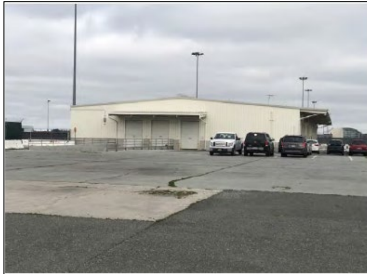
Photo 5. Air Freight Hangar – Belly Freight southeast elevation, view to the west
