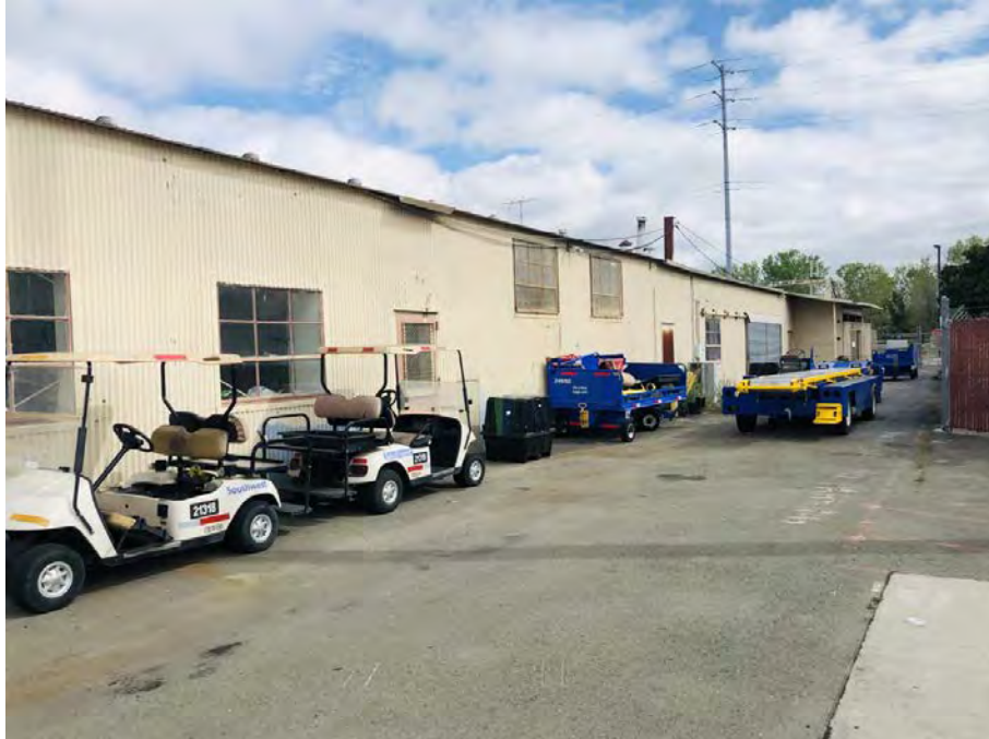
Image 31: Hangar 1253 southeast elevation, view to the northeast
