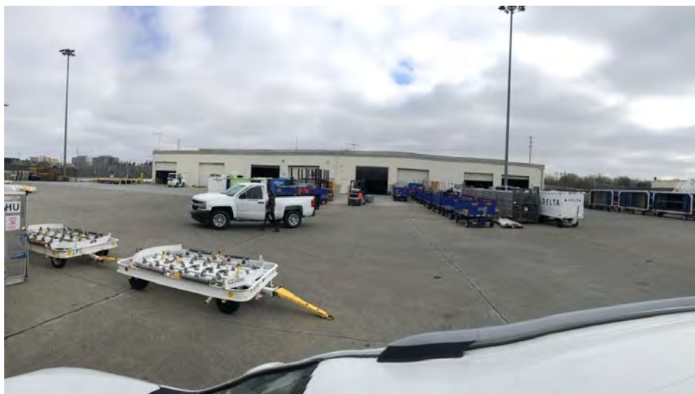
Image 11: Air Freight Building southwest elevation, view to the northeast
