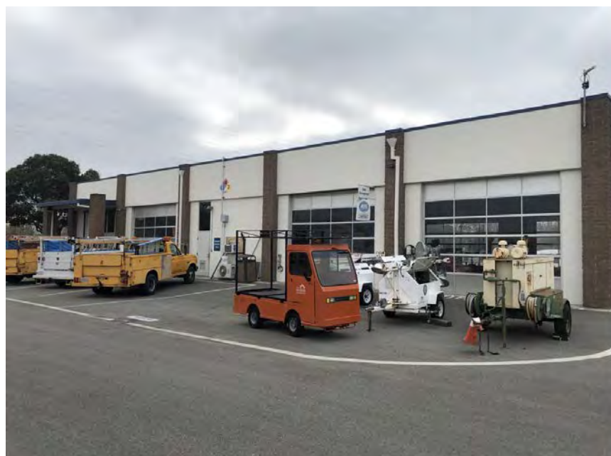
Image 18: Facilities Building (1395A) west elevation, view to the northeast
