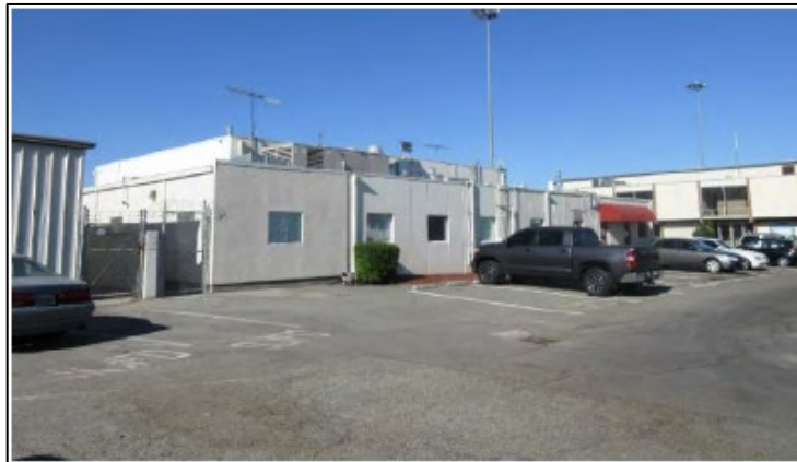
Photo 8. Aircraft Rescue and Firefighting Building northeast elevation, view to the west (Photo courtesy of the Evaluation of San Jose International Airport Aircraft Rescue and Firefighting Building Memorandum, 2018)
