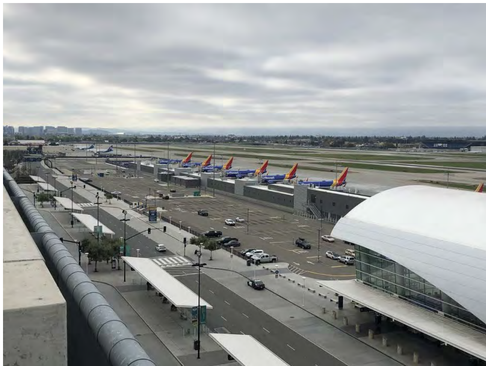
Image 45: Terminal B and surface parking, view to the south
