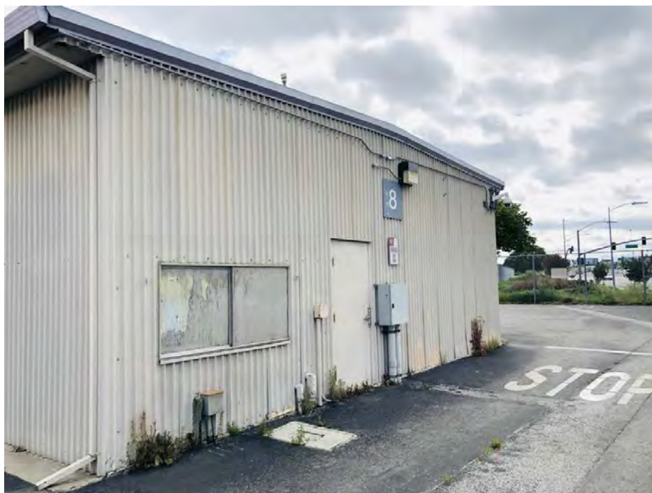
Image 35: Hangar No. 8 southwest elevation, view to the southeast
