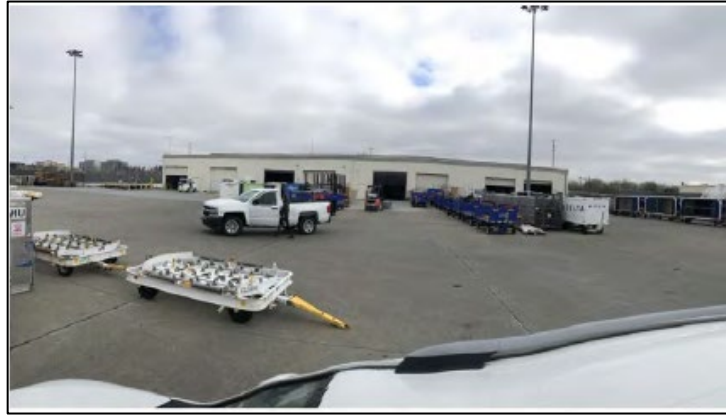
Photo 7. Air Freight Hangar – Belly Freight southwest elevation, view to the northeast
