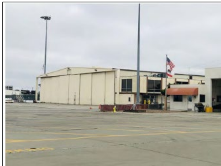
Photo 2. SJPD Hangar (ACM/Pestana) southwest elevation, view to the north
