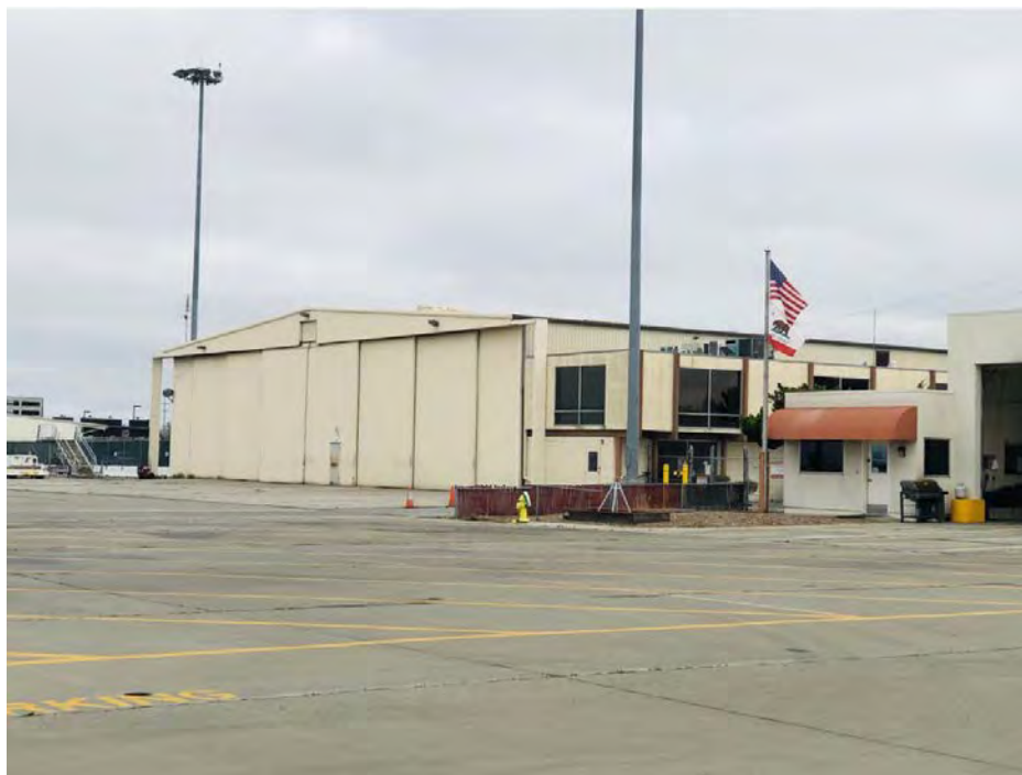
Image 13: ACM/Pestana southwest elevation, view to the north
