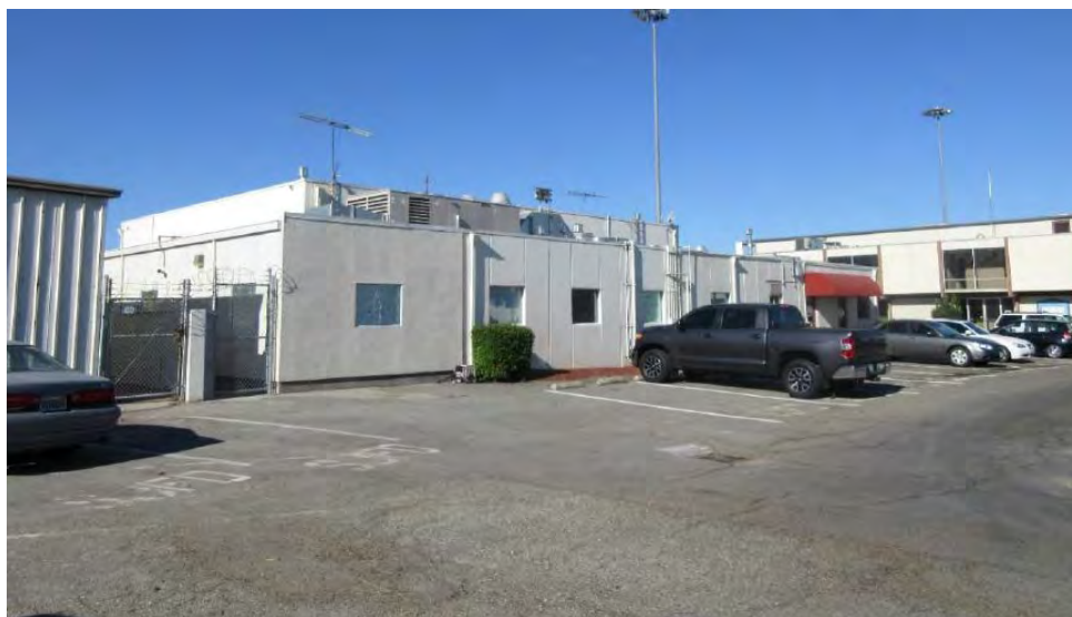
Image 16: Aircraft Rescue and Firefighting Building northeast elevation, view to the west
