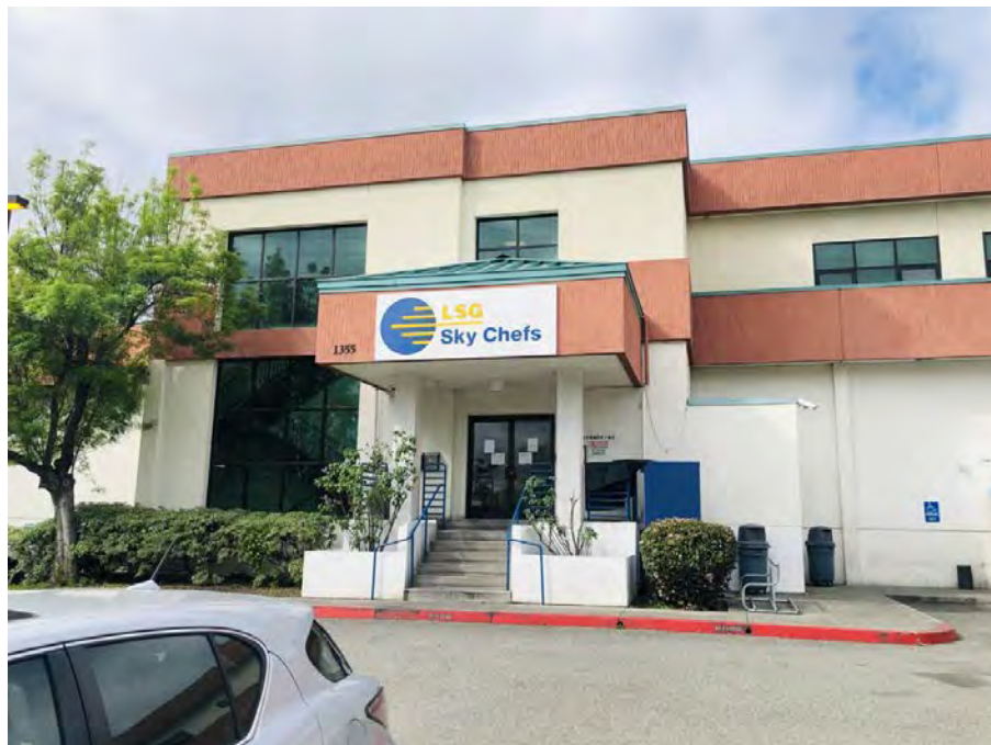
Image 22: In-Flight Kitchen northeast elevation, view to the southwest
