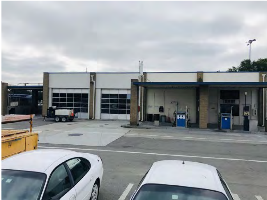
Image 21: Facilities Building (1395) west elevation, view to the east
