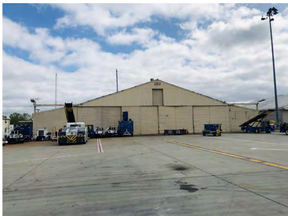
Image 30: Hangar 1253 southwest elevation, view to the northeast
