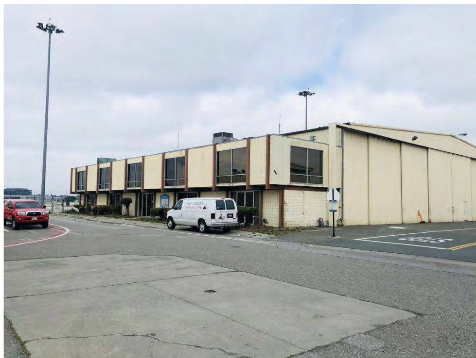
Image 12: ACM/Pestana Building southeast elevation, view to the northwest
