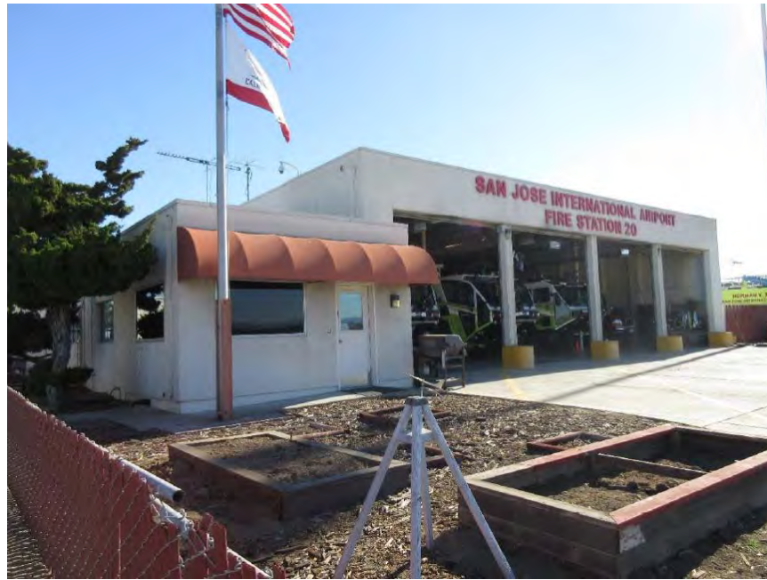
Image 17: Aircraft Rescue and Firefighting Building southwest elevation, view to the northeast
