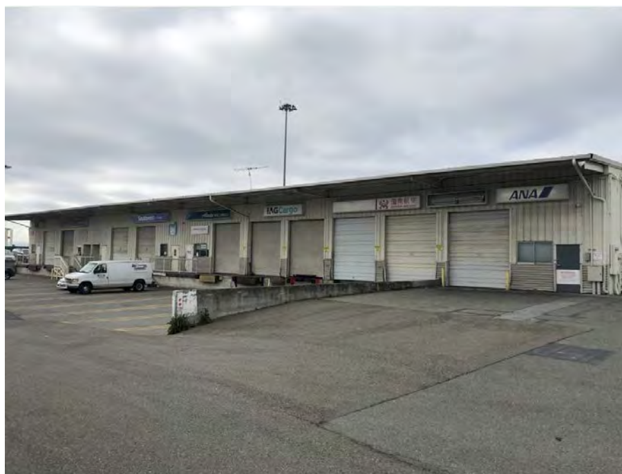
Image 10: Air Freight Building northeast elevation, view to the south
