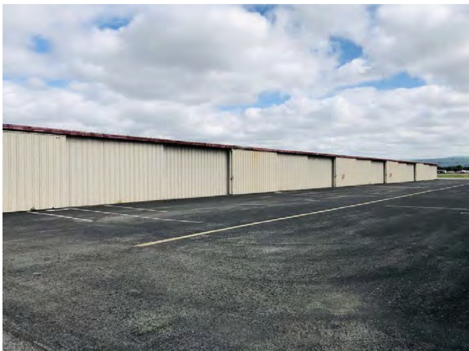
Image 36: Hangar 8 southeast elevation, view to the northeast
