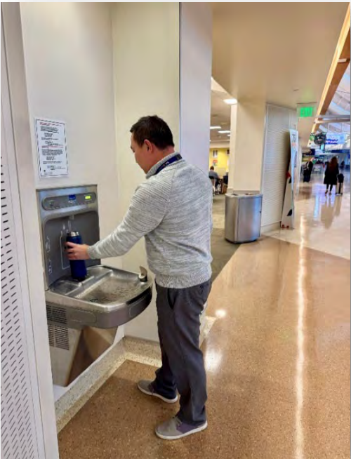
Water refill station in Terminal B.
